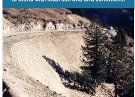
Erosion caused by sheet flow runoff evident on the area not stabilized by the GEOWEB material.
