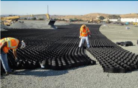
Installing 6 in deep GEOWEB sections over a woven geotextile & 2 in aggregate base
