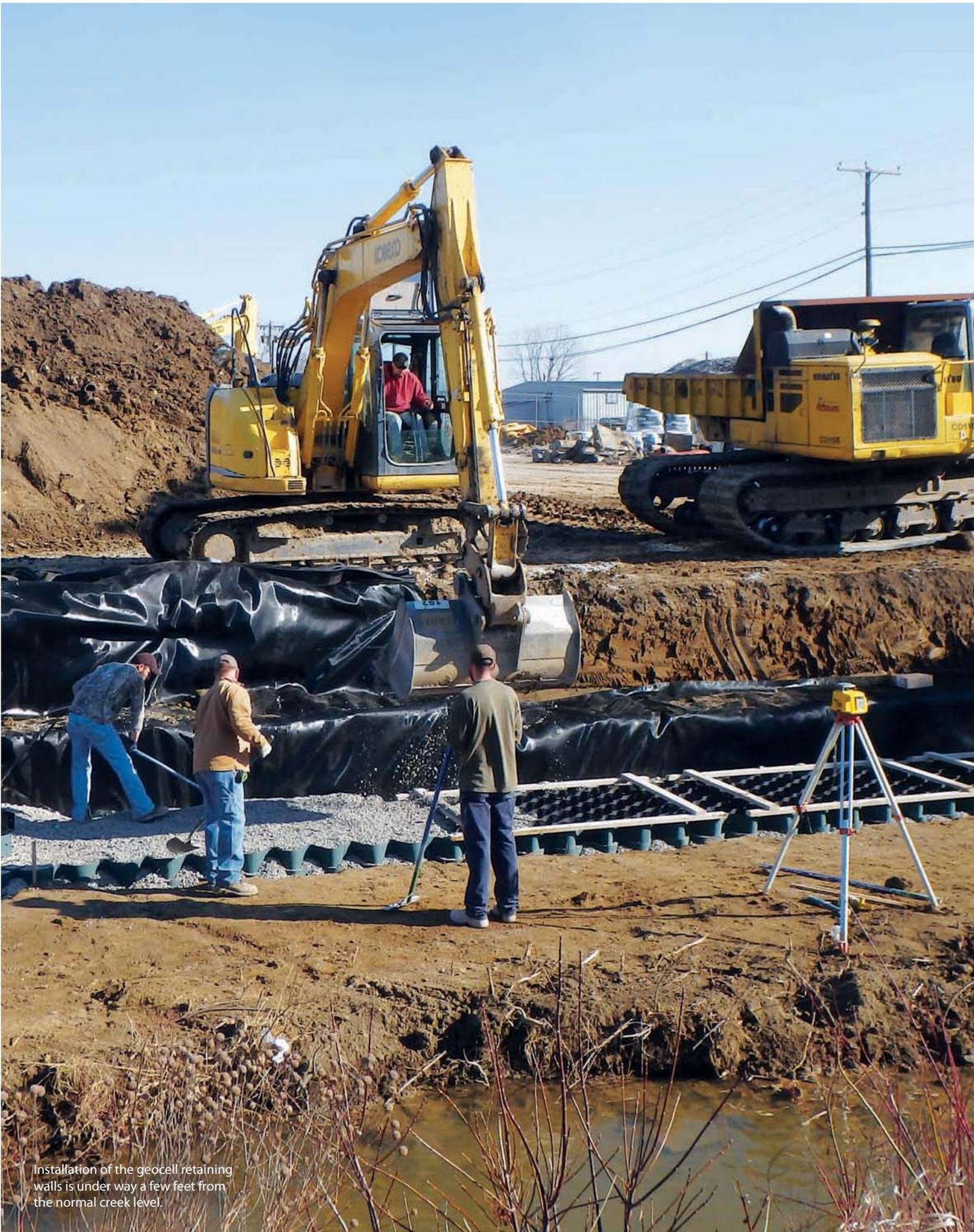
Installation of the geocell retaining walls is under way a few feet from the normal creek level.
