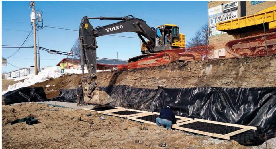
Wooden stretcher frames keep geocell wall sections open during infilling. Once filled the stretcher frames are removed and reused.
