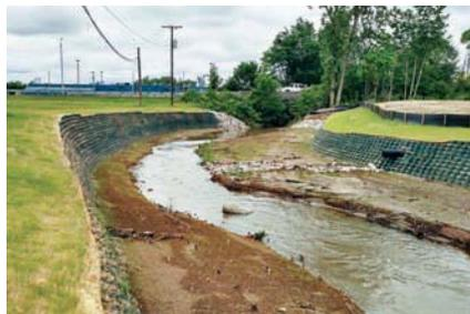
Completed geocell walls offer protection to an area of the watershed prone to flash flooding.
