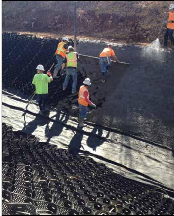
The 3D cellular structure holds concrete on the 1.5H:1V embankments.
