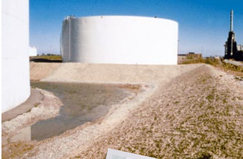
Completed concrete infilled Geoweb dike protection system.
