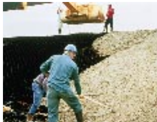
Application of concrete infill.
