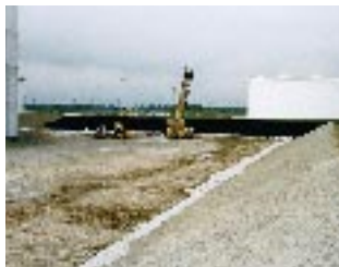
Geoweb panels conform to slope irregularities, improving quality and reducing infill waste.
