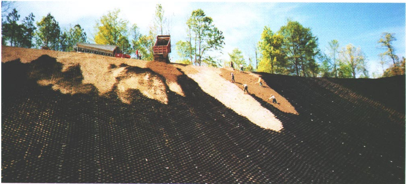
Photo 1. Infill is sprayed over the cellular-confinement system as installers rake the material into the cells.
