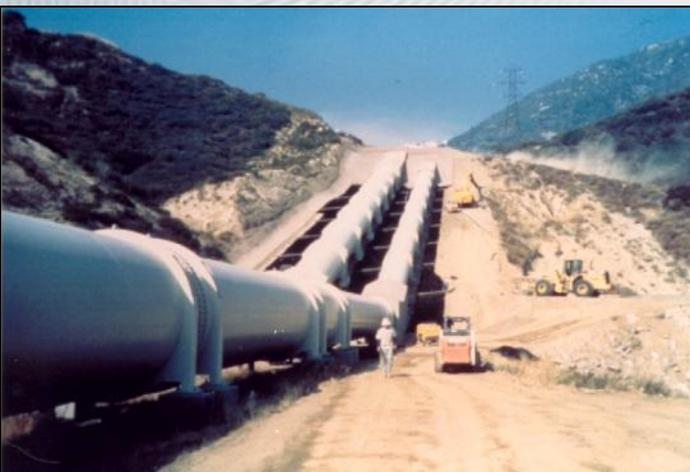
In 1994, the pipelines were in trouble. Erosion of the structures built to support the pipelines due to decades of water runoff was noticed. Winter was just around the corner and engineers looked for a solution before further erosion threatened the pipelines.
