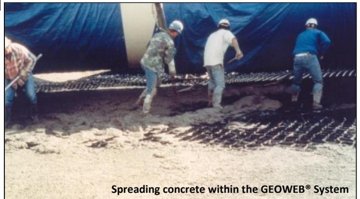
Spreading concrete within the GEOWEB® System
