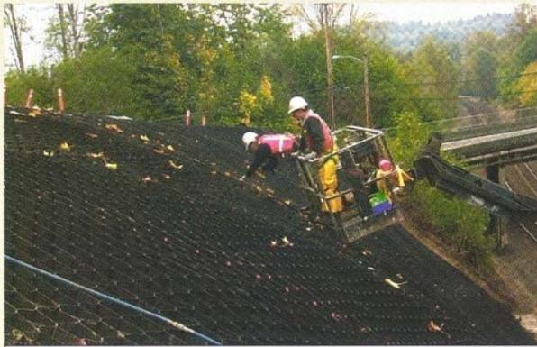
**Photo 4 (top).** To reduce erosion and the potential for sediment runoff to nearby salmon-bearing streams, no more than 40 ft. (12 m) of slope was left exposed after each work day.
