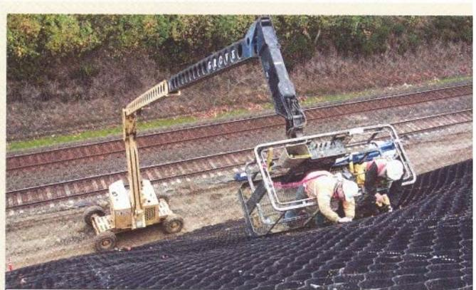
**Photo 3.** Following close upon the excavation crew's work, the installation team placed geotextile on the prepared slope face.
