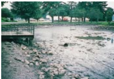
The drained pond prior to restoration.
