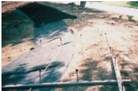
Wood templates facilitate positioning of anchors.
