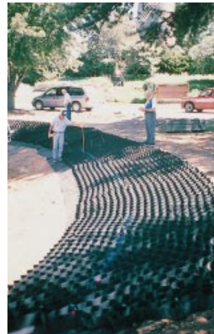
Geoweb® sections are ready for infill placement.
