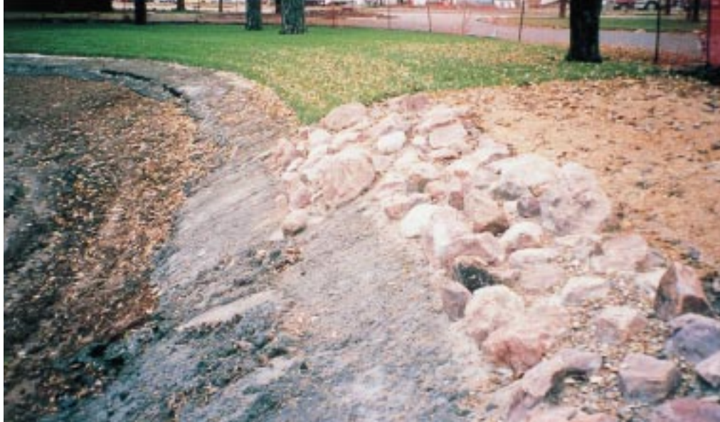
A rock garden effect is created by placing red granite within the concrete-filled system.
