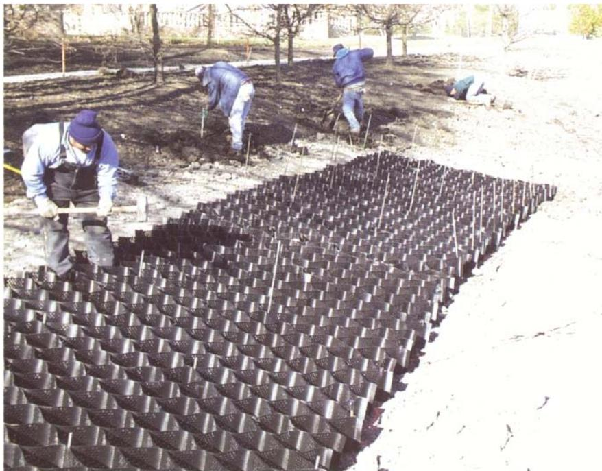
**Photo 2.** Geocellular systems are effective counters to shoreline erosion.
