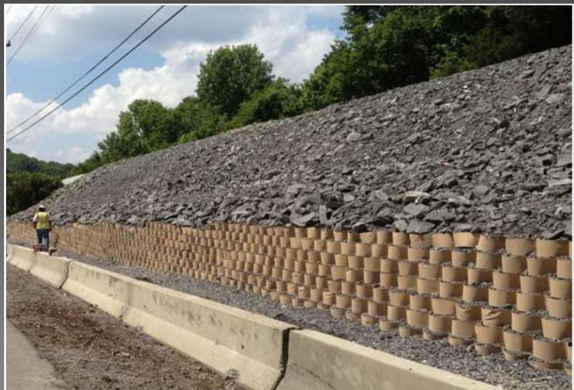
Completed GEOWEB retaining wall system with aggregate infill.
