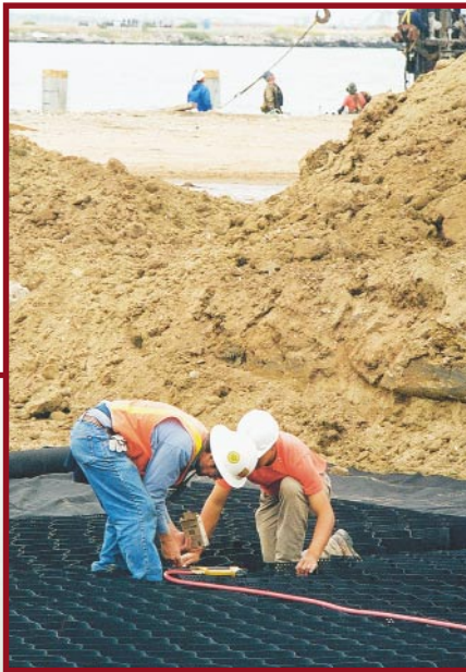
Some 213,000 square feet of GEOWEB was installed on the project.
