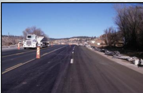
The finished roadway is paved with asphalt.
