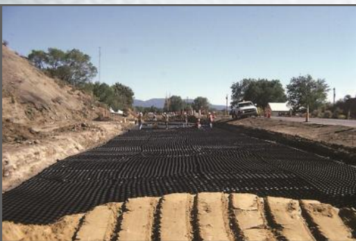
Infilling the GEOWEB sections with locally-available sand.
