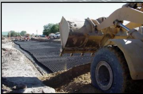
Dumping sand infill in the GEOWEB cellular confinement system.
