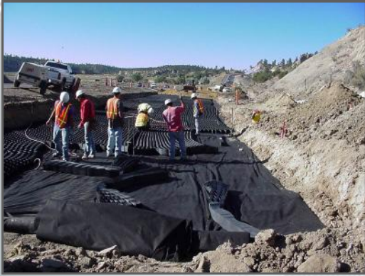
Expanding the GEOWEB sections over a geotextile.
