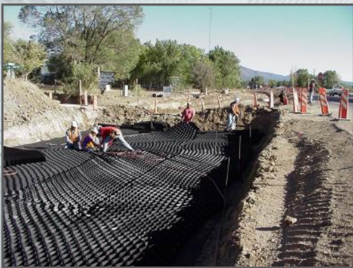
Connecting adjacent GEOWEB sections prior to infill.
