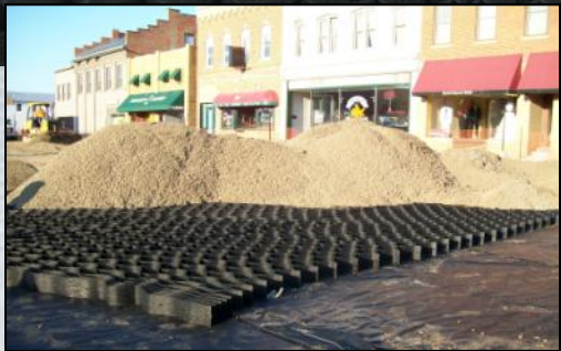
Aggregate ready to be spread in the GEOWEB® cellular confinement system.
