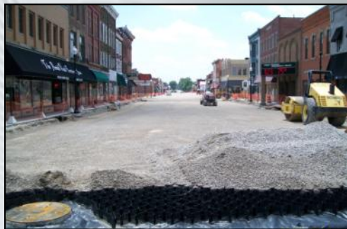
GEOWEB® system nearly filled with aggregate.
