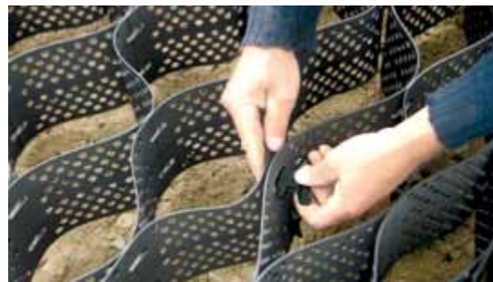
Connecting GEOWEB® sections with ATRA® Keys.
