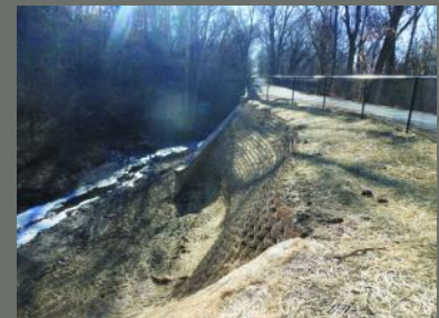
Completed GEOWEB wall section installed above a gabion base.
