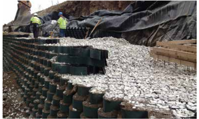
Construction of the Geoweb retaining wall system is performed in layers. A topsoil/aggregate mix is placed in the front cells to support vegetation and resist erosive forces. Aggregate is placed in the back cells to facilitate drainage.
