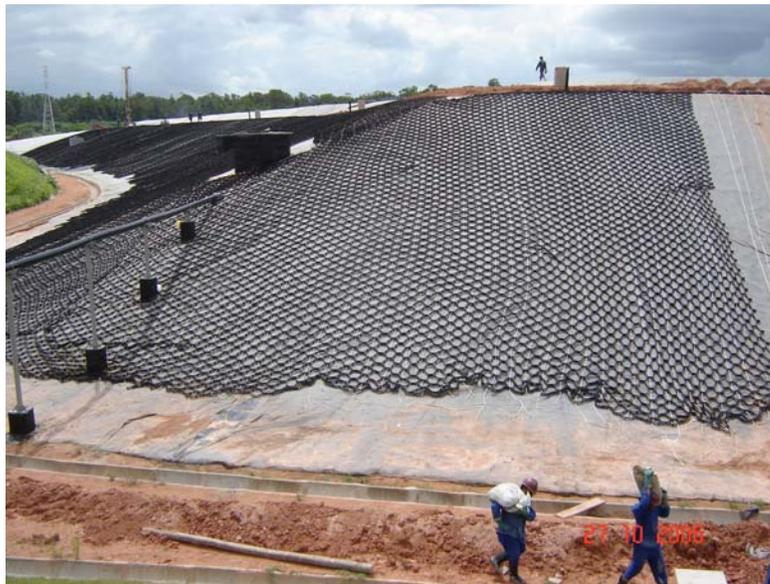
**Installation of the perforated Geoweb® sections over the textured geomembrane.**
