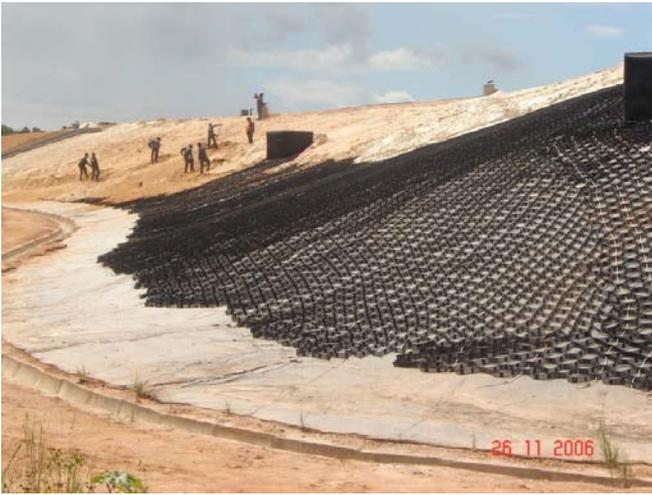
**Infilling the Geoweb system with sand.**
