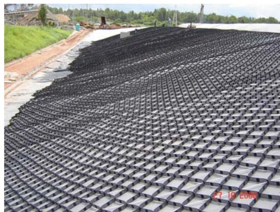
**Tendoned Geoweb sections installed and ready for sand infill.**
