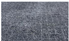
Placing and connecting the GEOPAVE with U-Clips, and infilling with crushed aggregate.
