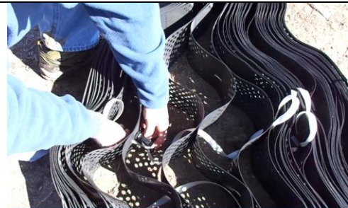
Figure 10 Preassembling ATRA Tendon Clips
