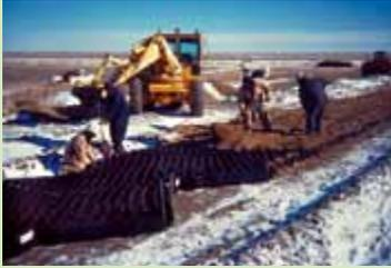
In load support applications, the GEOWEB® system generates powerful confinement forces and soil-to-cell wall friction creating a load dispersion structure with high flexural strength. The results, significant
